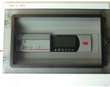
Wall Mounted Control Box
