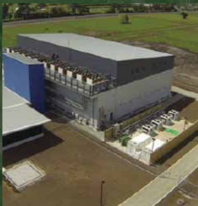
Spark Data Centre Auckland, New Zealand
